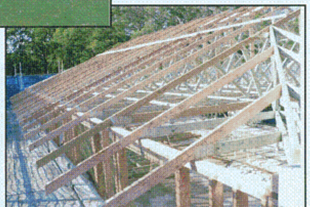
And in next to no time all the trusses are in place.
