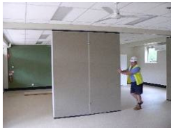
Paynter Dixon Site Manager for the construction of the new library and multi-purpose building, Kevin Hogg, demonstrates the operation of the
